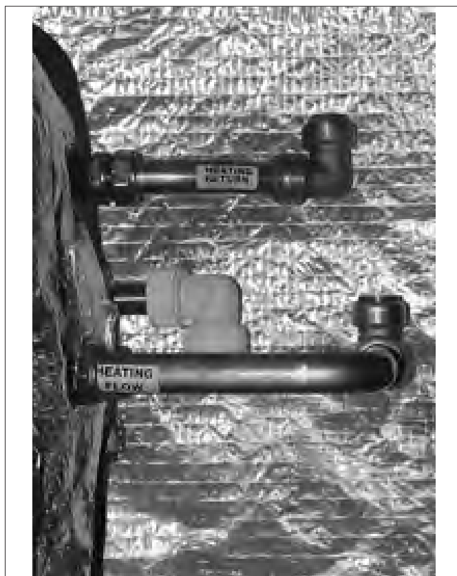
Figure 5-1: Non system boiler flow and return connections
