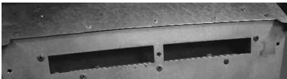
Fig 4 - Flue Restrictor Baffle Not Fitted
